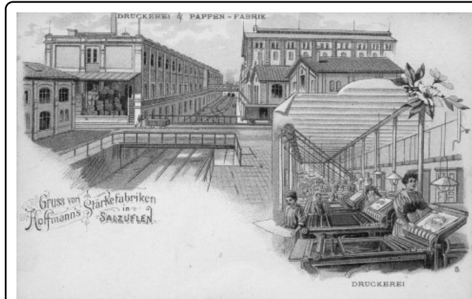
Greetings from Hoffmann's Stärkefabriken (starch works) in Salzuflen, Germany. This beautiful chromolitho card (card no. 5 in a series of?) of pre 1900 make shows a view of the own print works and board mill. Many bigger companies back then tended to have every production process inclusive their own (packaging/advertising) print shop within their walls. "Hoffmann" brand is still in business today.
